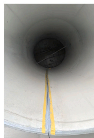
(c) Optical cable deployment
