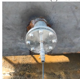
(b) Cable threading assembly
